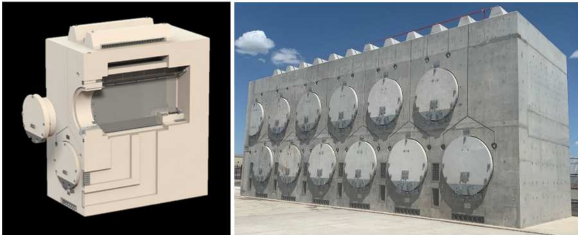
Fig. 48 Concrete casks Horizontal Ground-mount Type
