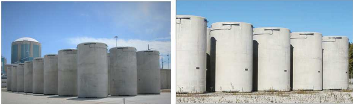
Fig. 46 Concrete casks Vertical Ground-mount Storage Type
