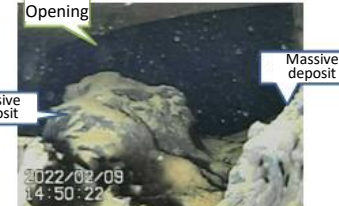
C. Inside of the pedestal opening
