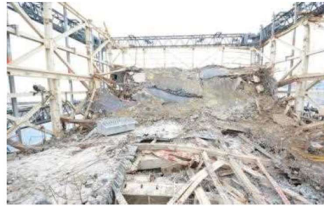
Condition of the collapsed south-side roof
