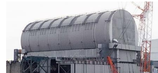
Cover for fuel removal was installed (Unit3) (Photo/video library:TEPCO)
