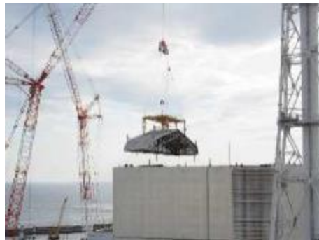
Removal of last one roof panel
