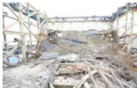
Condition of the collapsed south-side roof
