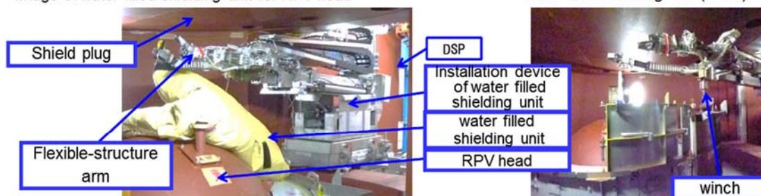
Installation device of water filled shielding unit
