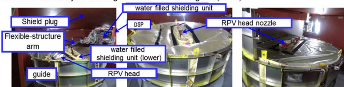
Installation of guide and water filled shielding unit
